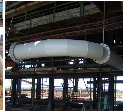
Concentrate receiving area
