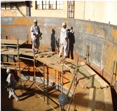
Tank rebuilding
