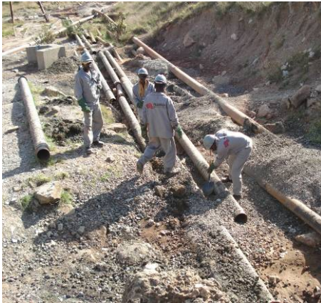
Pipeline replacement
