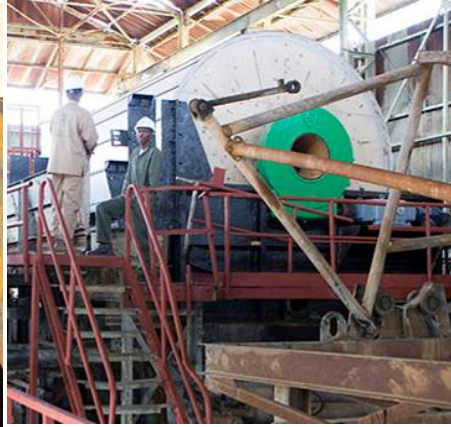
Drum filter repair
