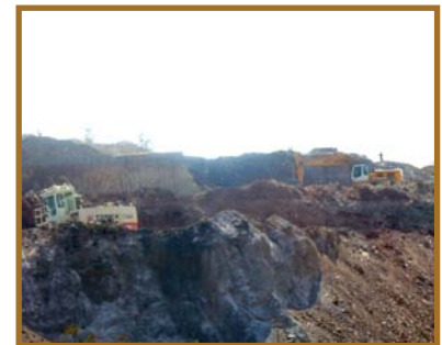
Pre-stripping at T17
