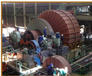
Final adjustments to mill no. 4
