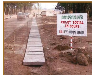
Concrete drain cover project
