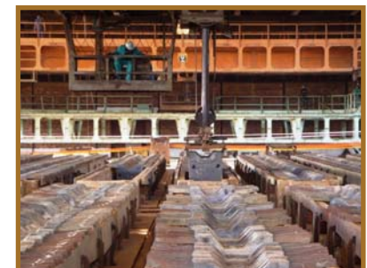
Lifting lead anodes at Luilu
