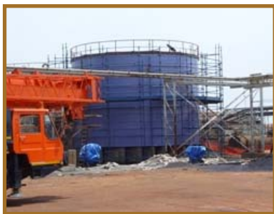
Acid tank construction
